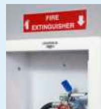
Safety labels ...and many more!
